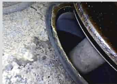
CLOSEUP OF THE HEALTHY O-320 exhaust valve, with a good view of the seat and valve-sealing surface.
